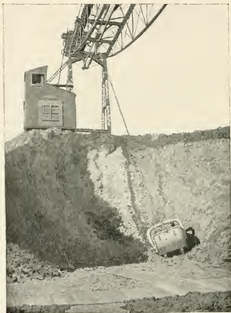
A Shovel-bucket in Use at the American-built Storage and Rehandling Plant at Mariupol, Russia.
